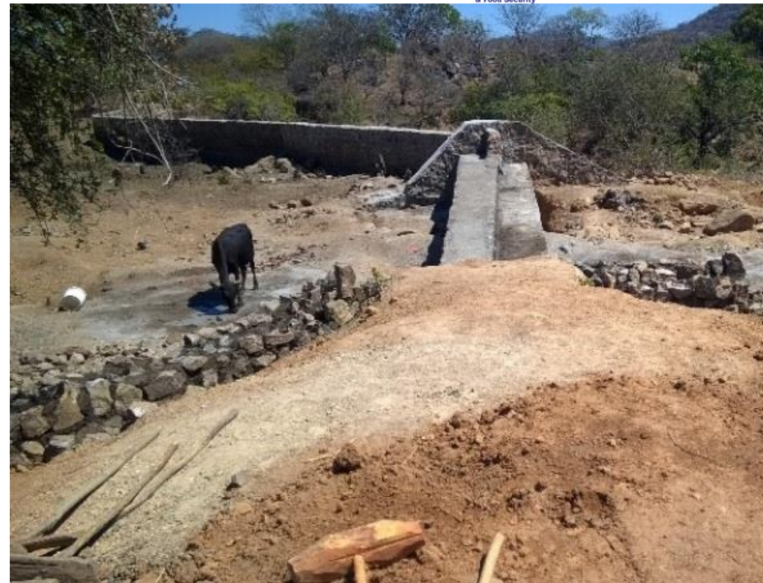
Figure 2. Nhora weir rehabilitation in 2016
