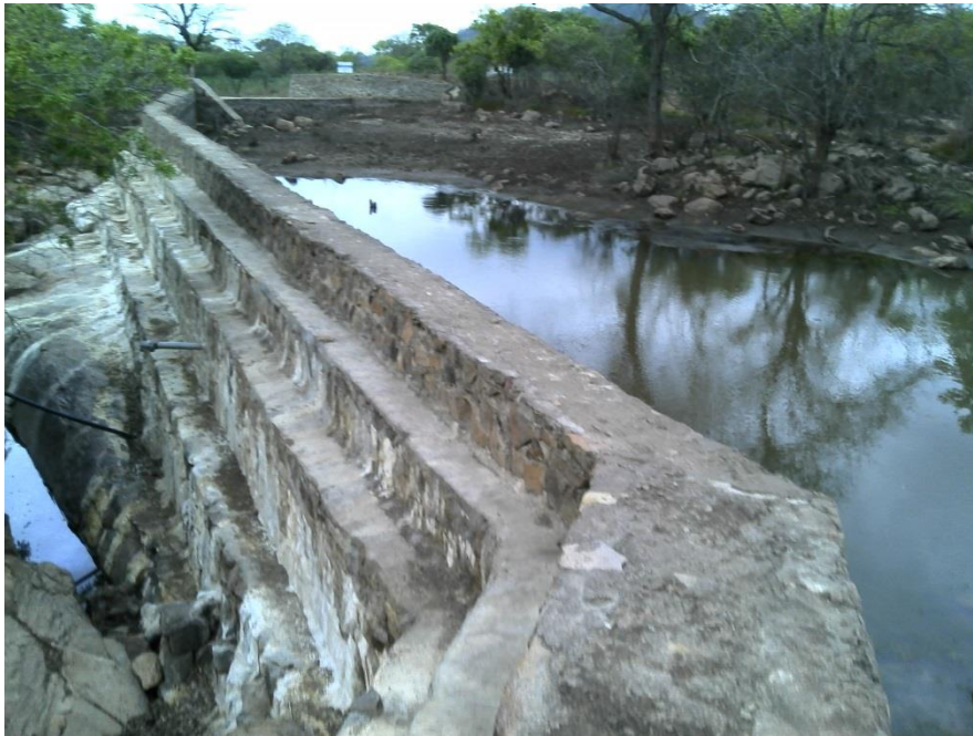
Figure 3. Nhora weir at 20% capacity October 2017
